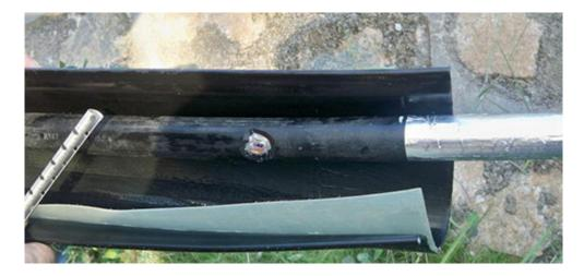
CRS Wraparound sleeve is mainly used for repairing outer/inner sheath/core damages on a HV cable and LV cable. It is made from cross-linked polyolefin which equals or exceeds the material properties of the original cable jacket. They can also be used for protecting against corrosion on metallic parts of the cable that are exposed to the outside.
